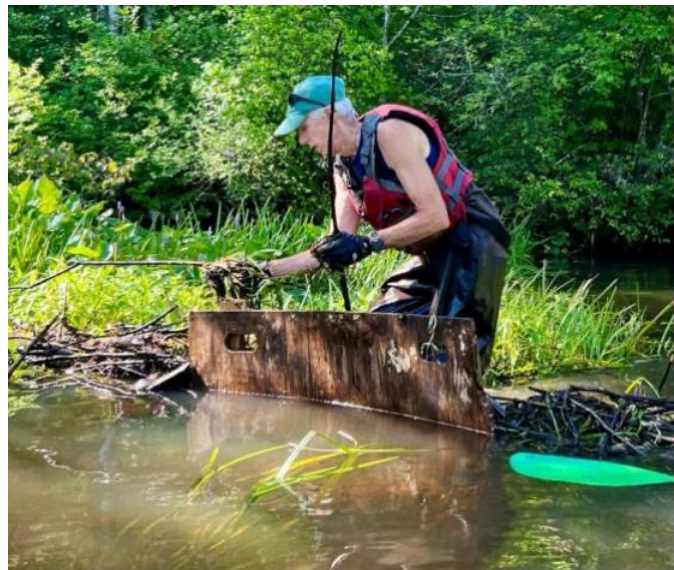
Jack Installing the gate and weaving sticks back into the dam.
